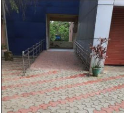
Ramp Facility at RC Bhubaneswar
